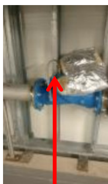
EPDM flexible hose to dishwashers
