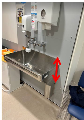
Figure 54. Excess splashing due to deep trough sink
