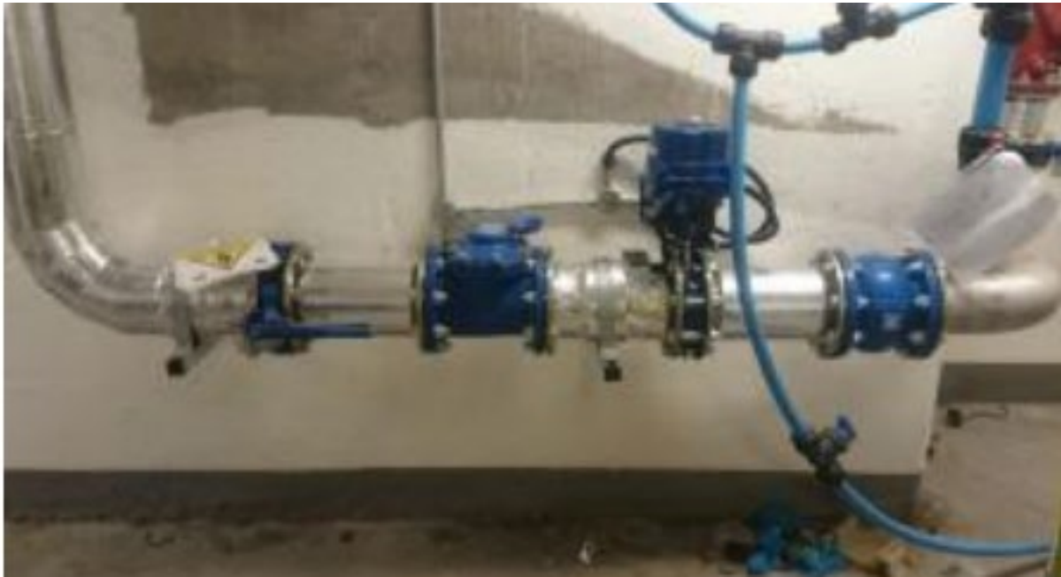
Figure 4. Hardgate mains water supply Image 93 .
