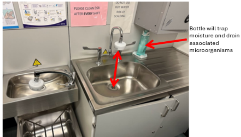
Figure 55. Excessive splashing of drain related microorganisms and inappropriate storage of items on sink.
