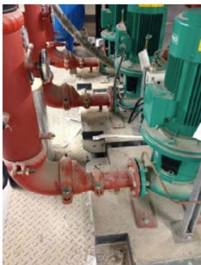
Figure 33: Low Temperature Hot Water (LTHW) pumps 150
