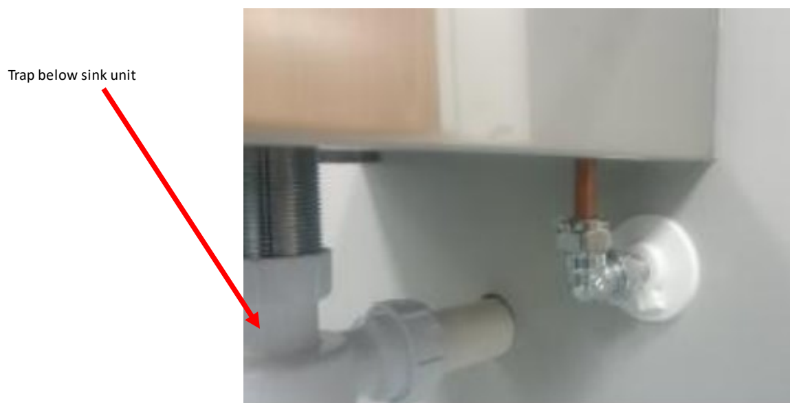
Figure 23. Position of trap below a sink unit.
