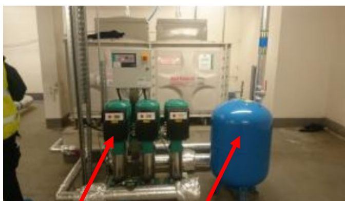
Trade booster pumps (green) with manifold and expansionvessels (blue)– source DMA L8 RA VT2.0
